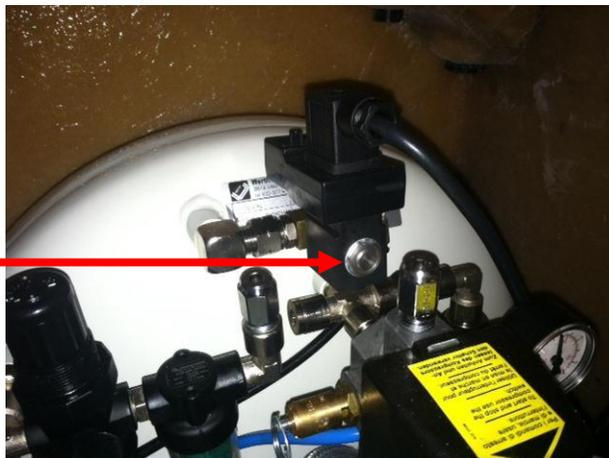
4. Once the silver hex nut is removed and the control module box is loose, you will be able to slide the Auto Drain control module box forward. Unscrew the hex nut on the end/base of the brass bar where the control module box rest on.
